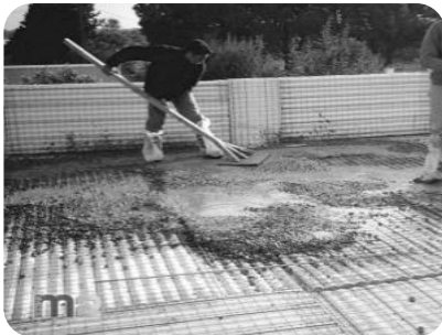
Accessible flat roof
